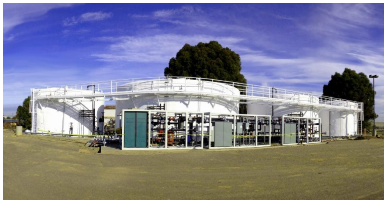
CleanWorld's Sacramento Biodigester when expanded will convert more than 37,000 tons of food waste per year into natural gas, electricity and soil-amendment products.
